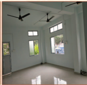
NE corner of meeting room
