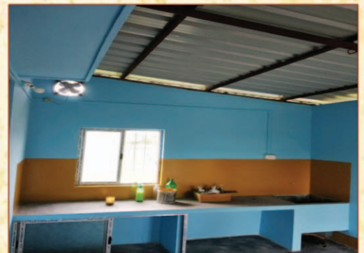
Kitchen of Grade IV quarter
